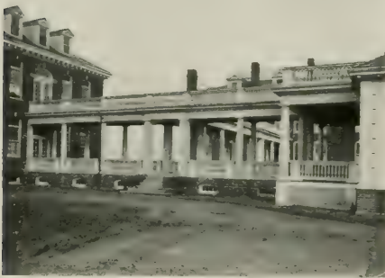
Fig. 3. Jordan Hospital. A connecting corridor.
